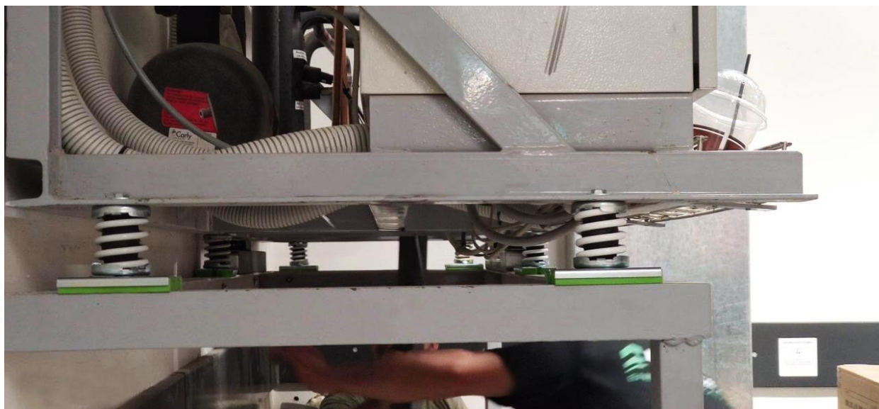
Primena vibroamortizera AMC Medium Series
