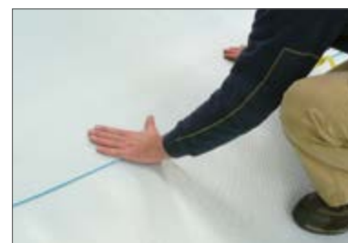
(3) Stick correctly the two layers together
