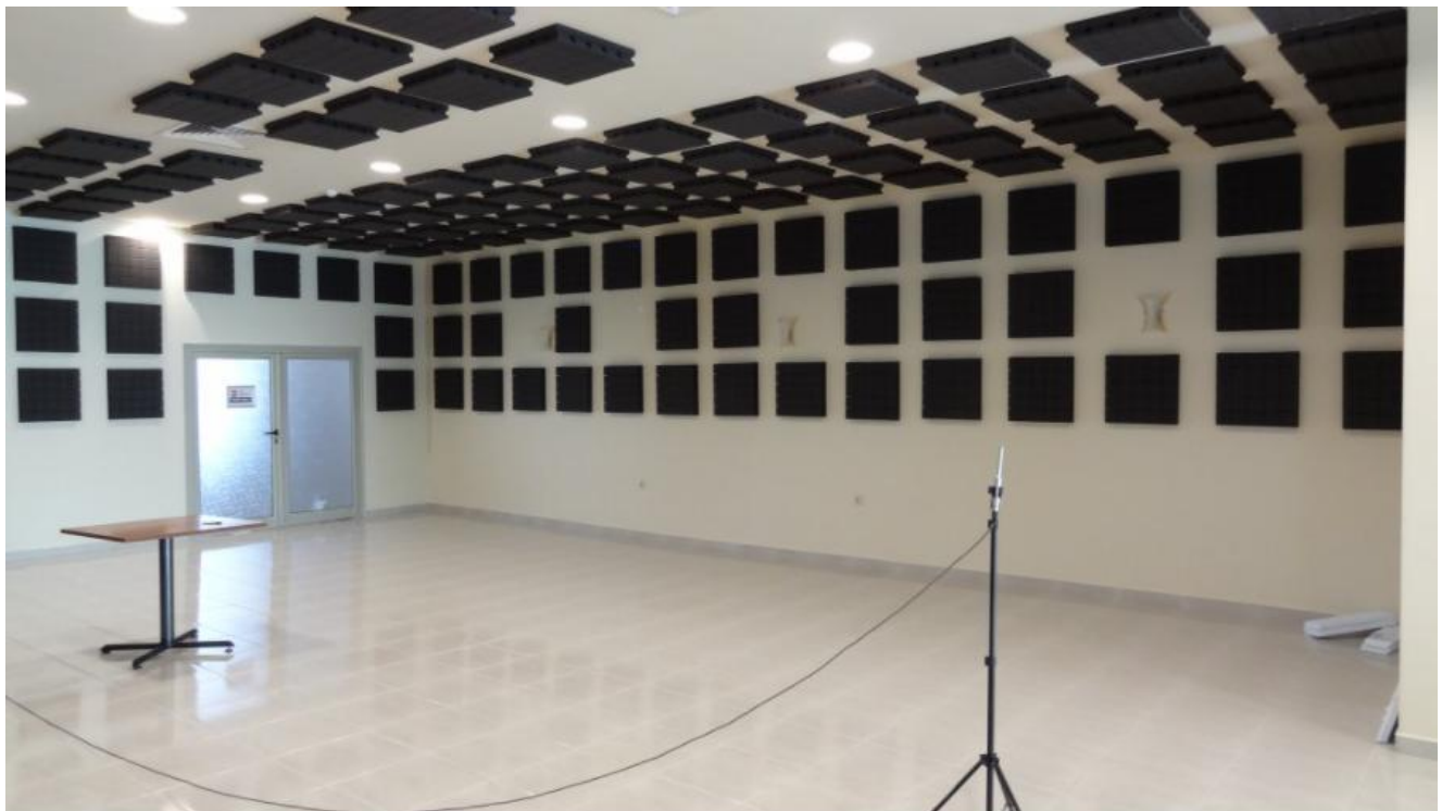
Primena panela Square raster apsorber
